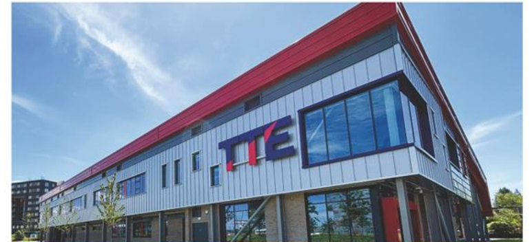
State-of-the-art £35m Engineering Technical Training Centre
