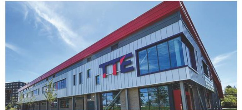
State-of-the-art £35m Engineering Technical Training Centre
