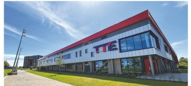
State-of-the-art £12m Engineering Technical Training Centre
